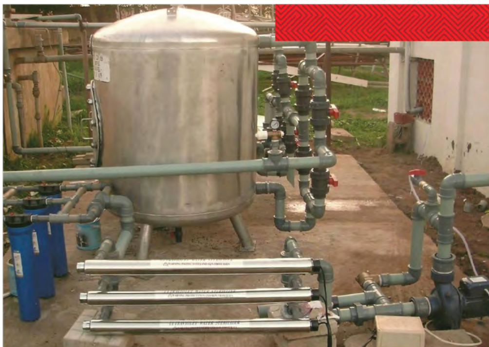
Construction of Solar Boreholes And Renovation of Reservoir, Adamawa State.
