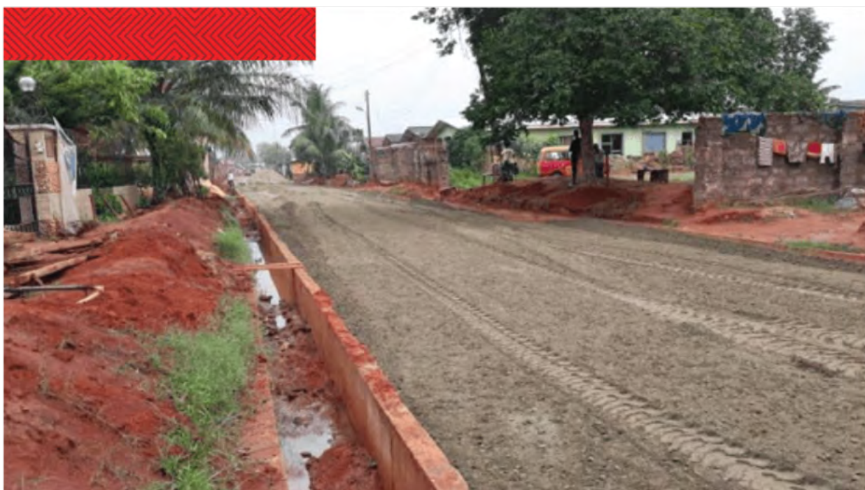
Construction of Uyo township roads [drainages], Akwa Ibom State.
